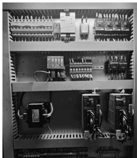
Figure 5 Internal structure of control box
